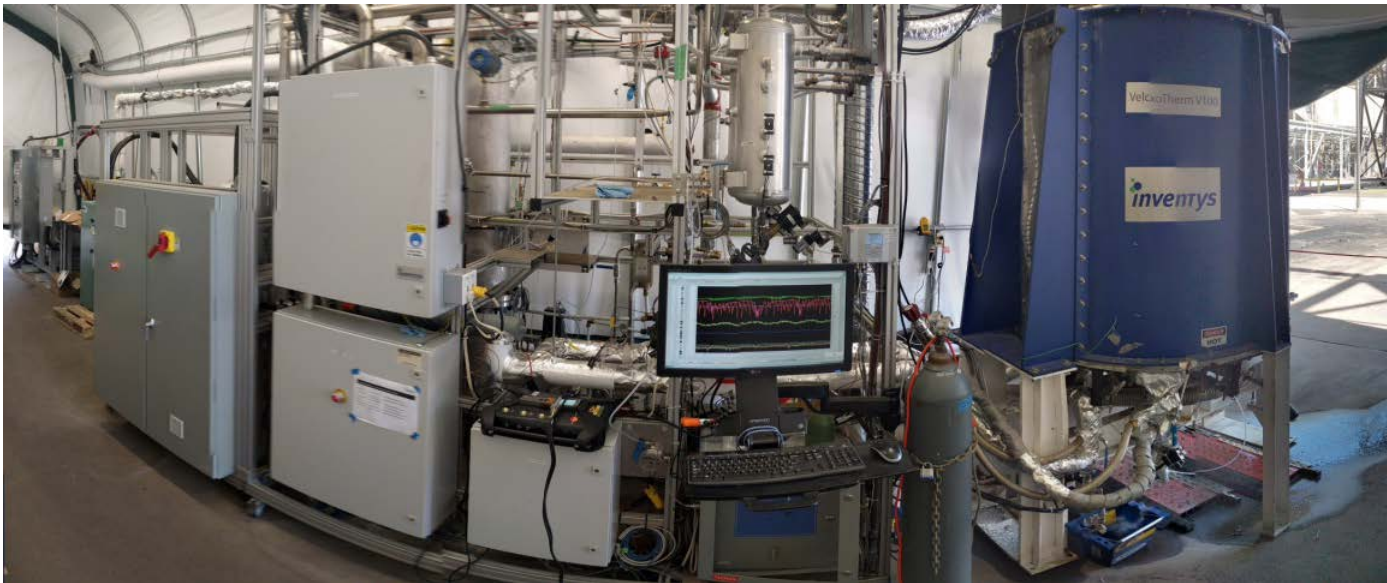
Inventys capture system operating on coal flue gas slipstream at NRG Parish
